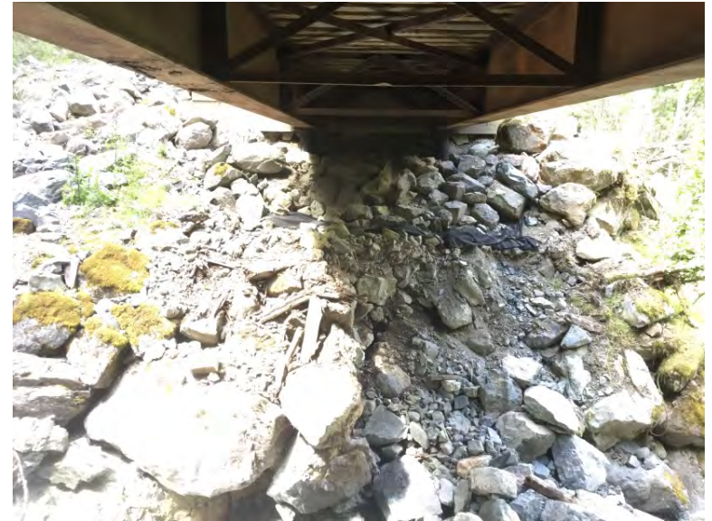
Left Bank Abutment when facing downstream
