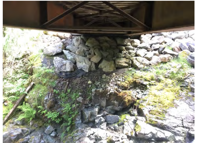
Right Bank Abutment when facing downstream
