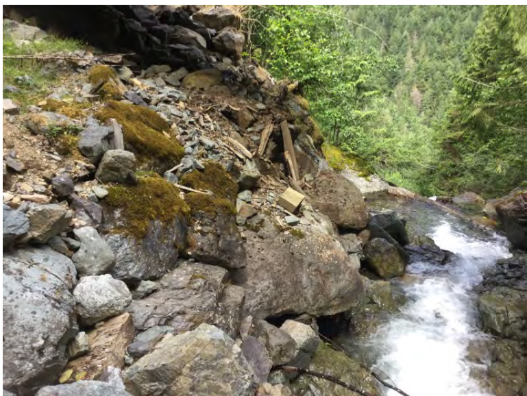
Upstream portion of left bank riprap
